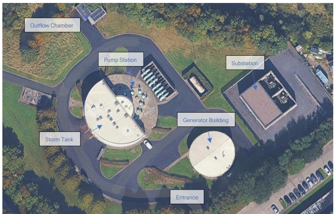
Figure 04: Existing Corcanree PS
